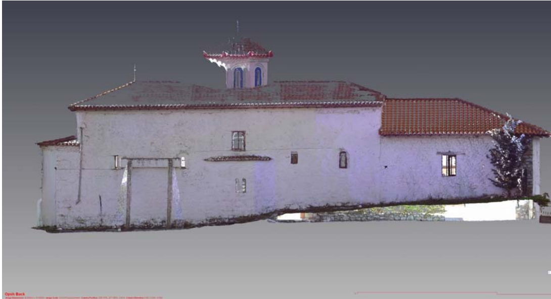
Fig. 4. Orthoimage of the north facade
